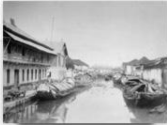
Canal in Binondo, ... Alexander Turnbull Library
